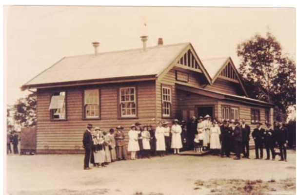
Opening of second room in Hallam Road School, February 1921 Source: Casey-Cardinia Local History Archive Collection
