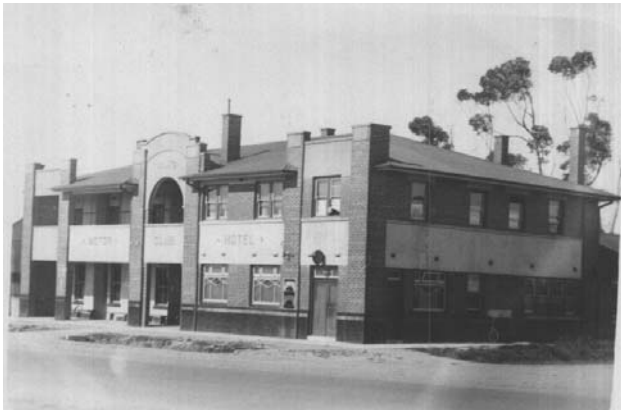
Kelley's Hotel, High Street Cranbourne, 1920s Source: Cranbourne Shire Historical Society
